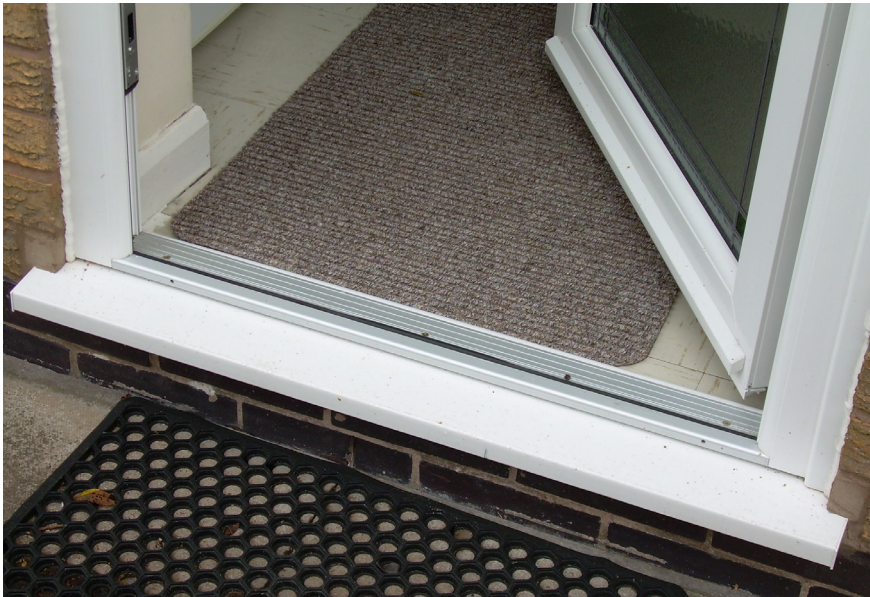
Low Aluminium threshold - reducing step-over height (ask for more details)
