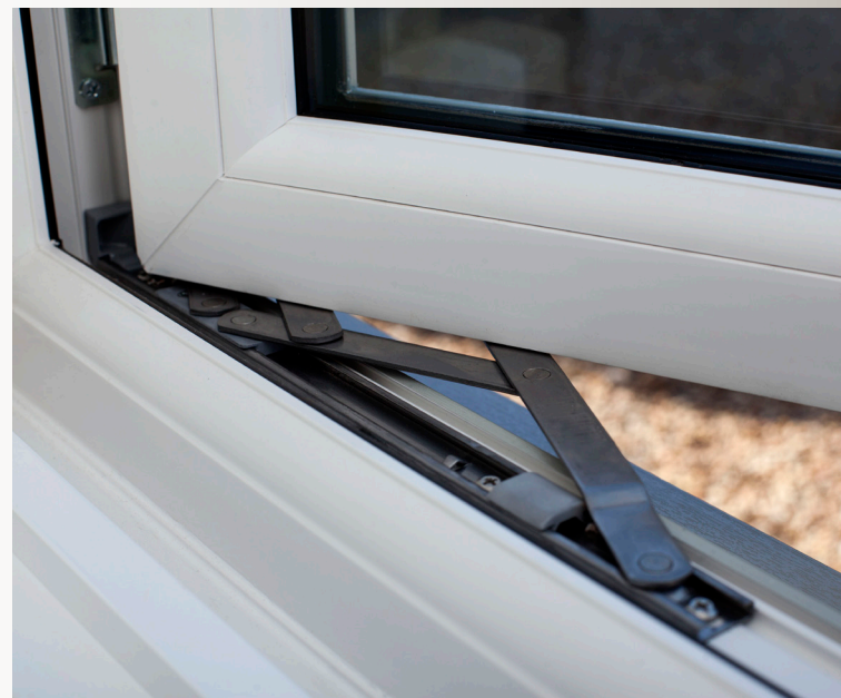
Close up of Sculptured Casement highlighting the Anti- Salt Egress Easy Clean Hinge
