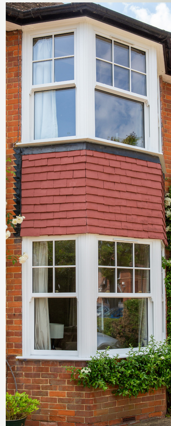
Bay Window fitted Using Vertical Sliders with Astragal Bars in the top Sash
