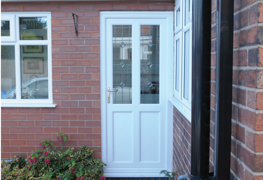
Residential Front door with Crucifix style Transom and Mullion with decorative glass and panel bottoms in White
